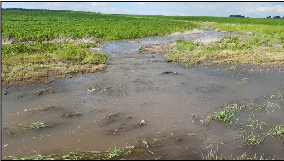
160 th St SW crossing of Browns Creek July 27, 2016
